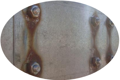
Mixed-material galvanic corrosion
